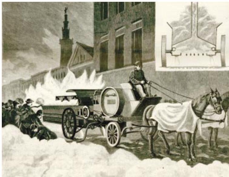
Snow-melting machine in operation
